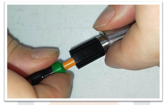
Screw the packing nut all the way until its fully inserted. Use spanners to ensure its fully secure. Failure to do so will result in possible water ingress.
